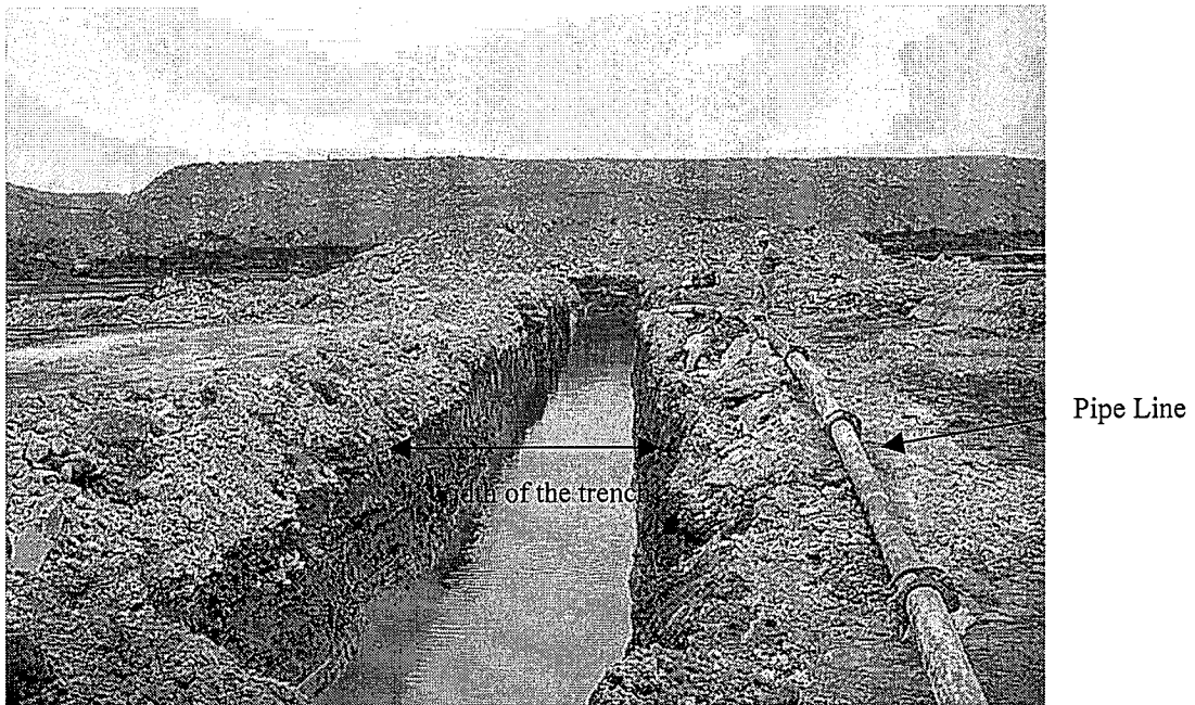
Figure 12B. Picture of the surface trench.
