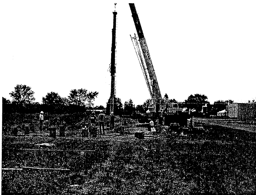
Figure 4. Pile Driving in Progress
