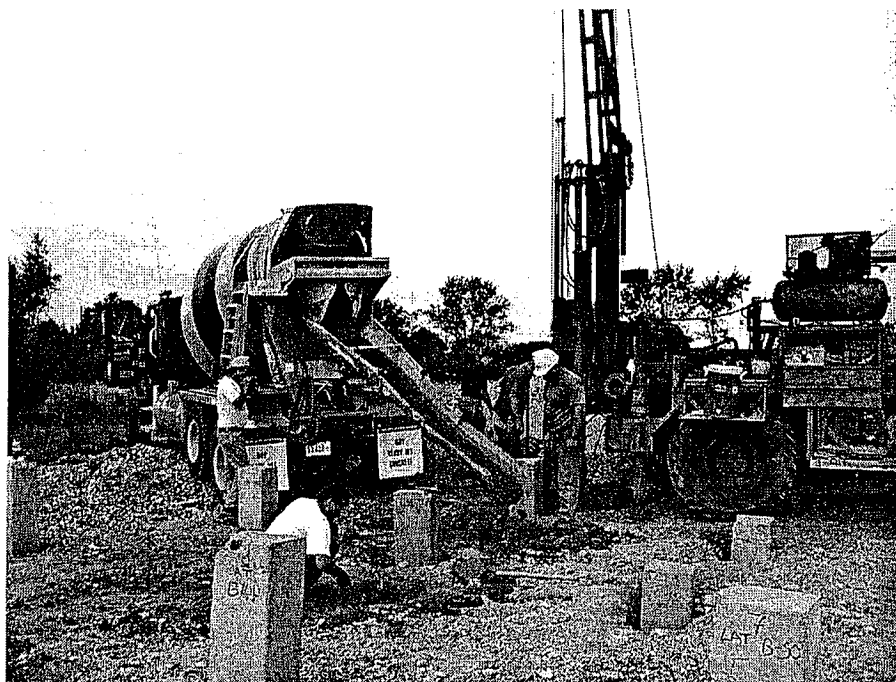
Figure 5. Construction of Reaction Piles in Progress
