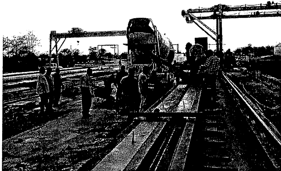
Figure 3. Pile construction in Progress
