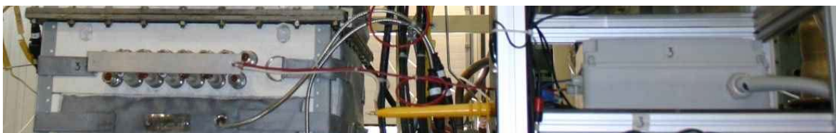
Figure 21. Power Modules Installation and Connection
