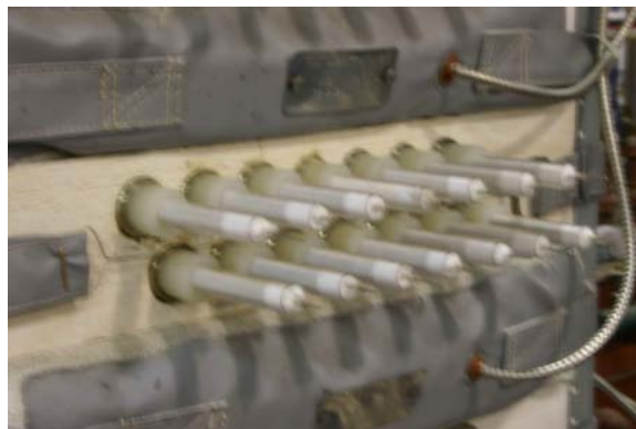
Figure 10. HV Electrodes Installed into the Reactor
