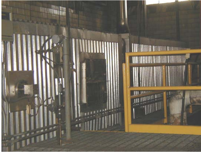
Figure 10: The location of the slipstream in the SIUC physical plant
