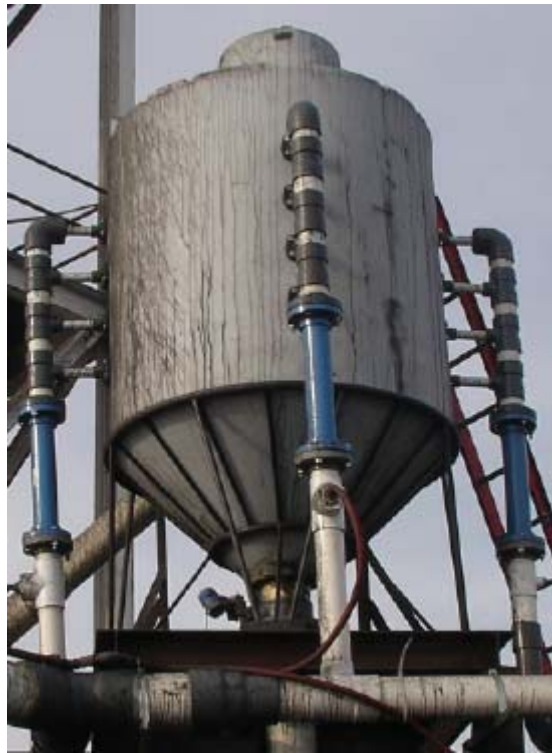
Figure 1. View of MRC (Providence One Installation) Showing Feed Input Arrangement
