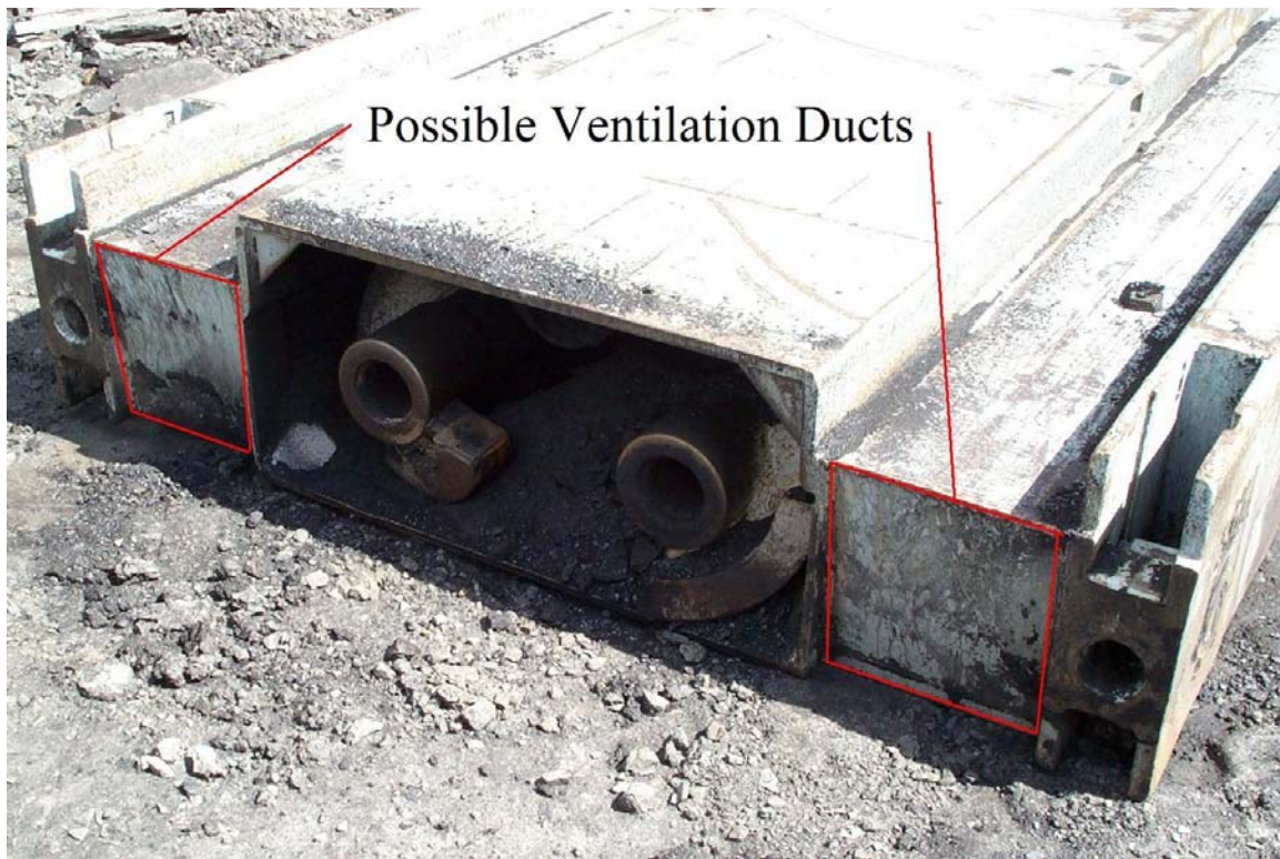
Figure 2. Push Beam with Possible Ventilation Duct Identified.
