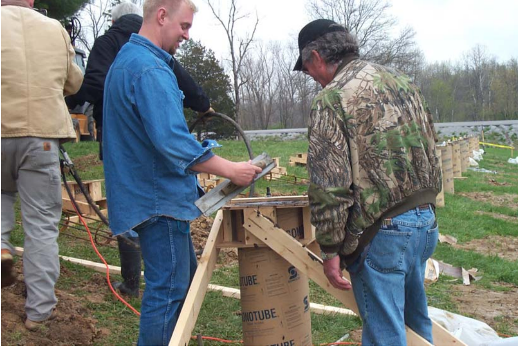
Figure 7. CCBs based foundation pier being finished after being poured.
