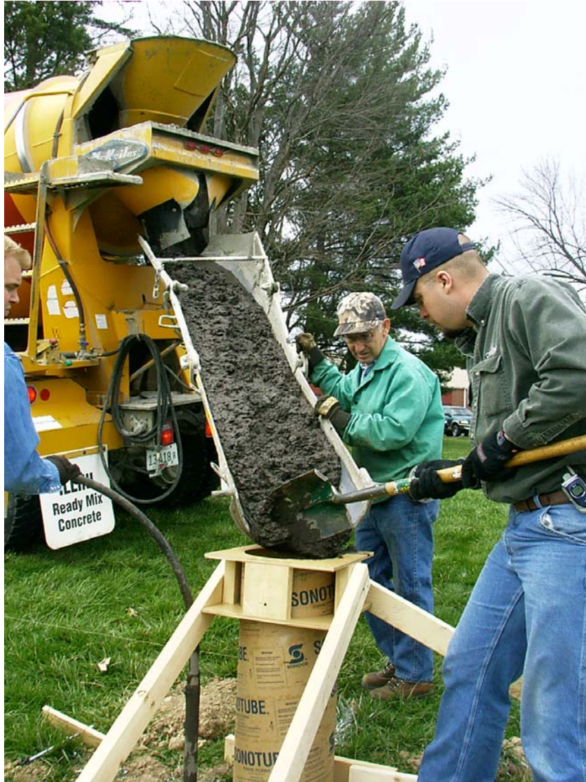
Figure 5. CCBs based foundation pier being poured.
