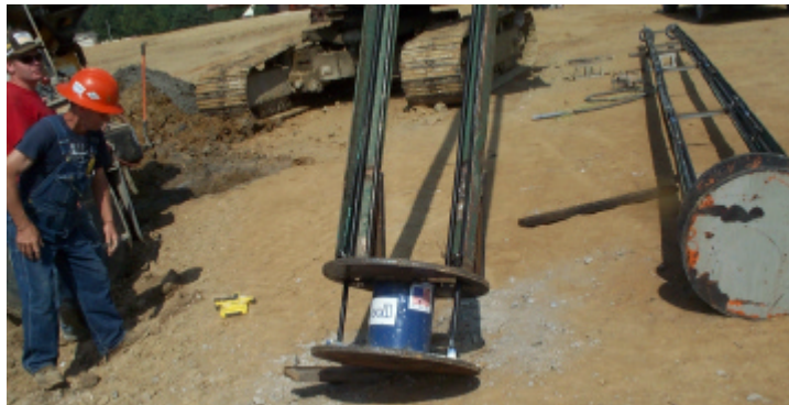
Figure 4. O-Cell attached to the steel frame and steel plates
