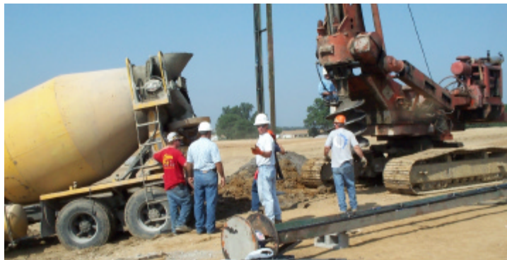
Figure 5. Construction of shafts in progress
