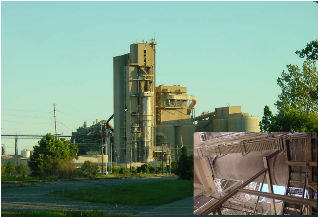
Figure 1. Cape Girardeau Cement is a Preheater-Precalciner Kiln Plant (Inset showing the rotary kiln)
