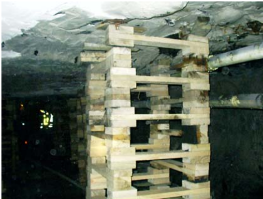
Figure 9: Installed ATLAS crib.
