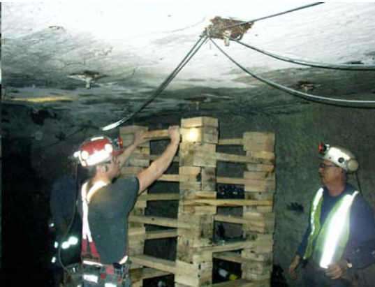
Figure 10: Installing an ATLAS crib.
