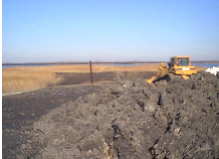
Figure 6. Dredging of prep-waste from slurry #2 pond
