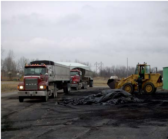
a) Prep-waste being loaded on trucks
