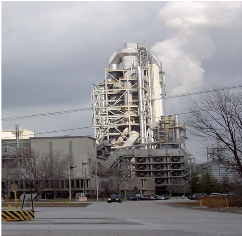
Figure 10. Greencastle Cement plant showing precalciner/preheater tower
