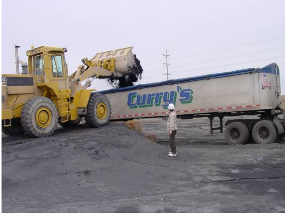
c) Prep-waste loading into trucks
