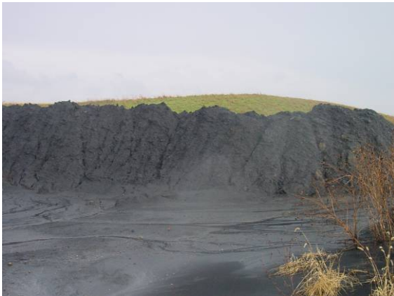
a) Prep-waste dredging and spreading
